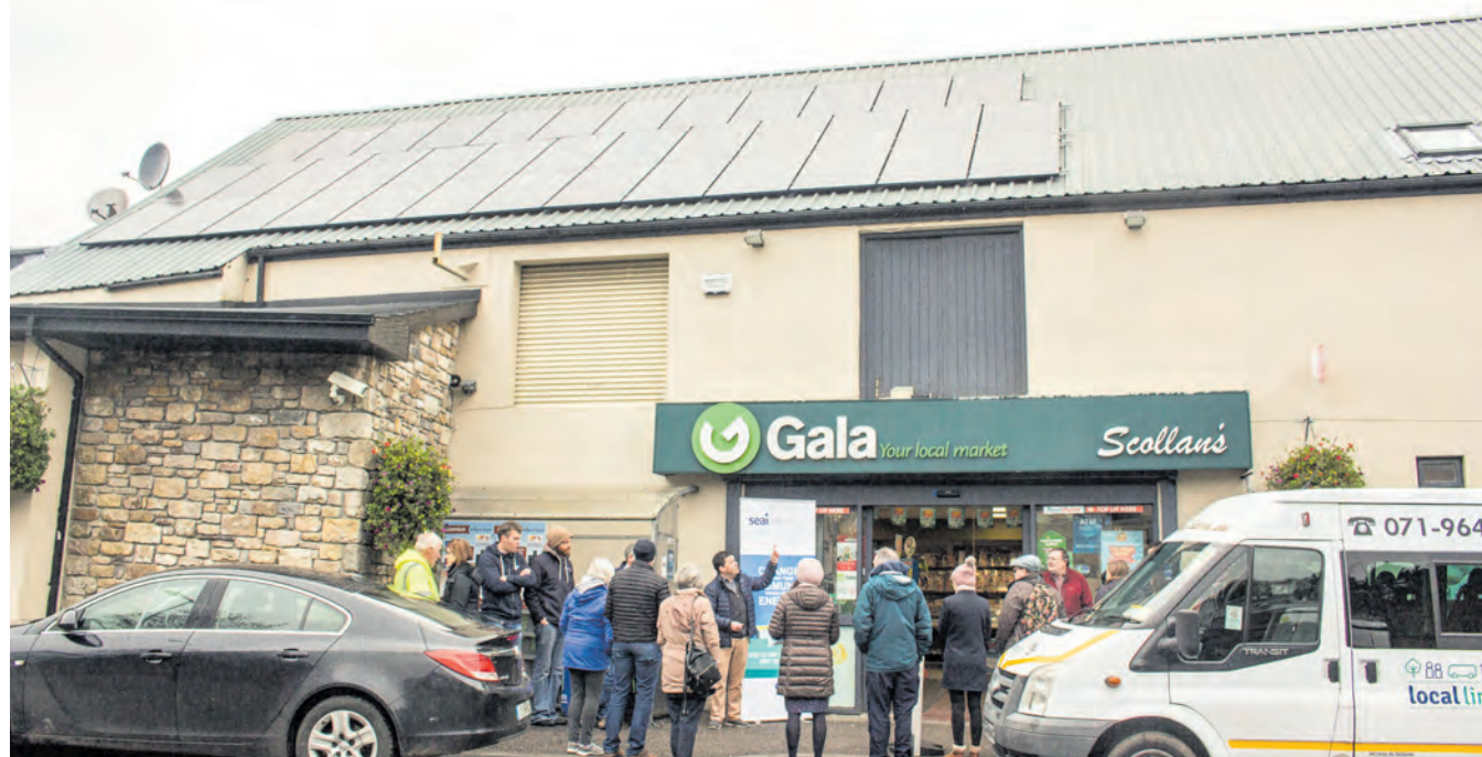
Pictured above is the 10 kWp Solar Photovoltaic system providing renewable electricity to the Scollan's Gala Superstore in Drumshanbo, Co. Leitrim producing approx 10,300 kWh/year.
