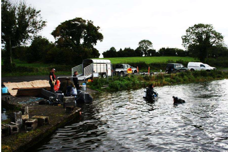
Plate 2. Scuba divers preparing to secure the jute mats on the lake bed and to stitch the layers together.
