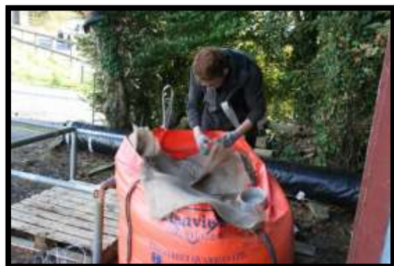
Plate 3.5 Preparing jute sheets from the mother roll for deployment in the lake, while weights of pea gravel and jute are prepared to hold the jute mat in place on the lake bed.
