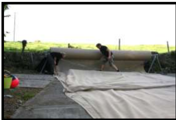
Plate 3.5 Preparing jute sheets from the mother roll for deployment in the lake, while weights of pea gravel and jute are prepared to hold the jute mat in place on the lake bed.
